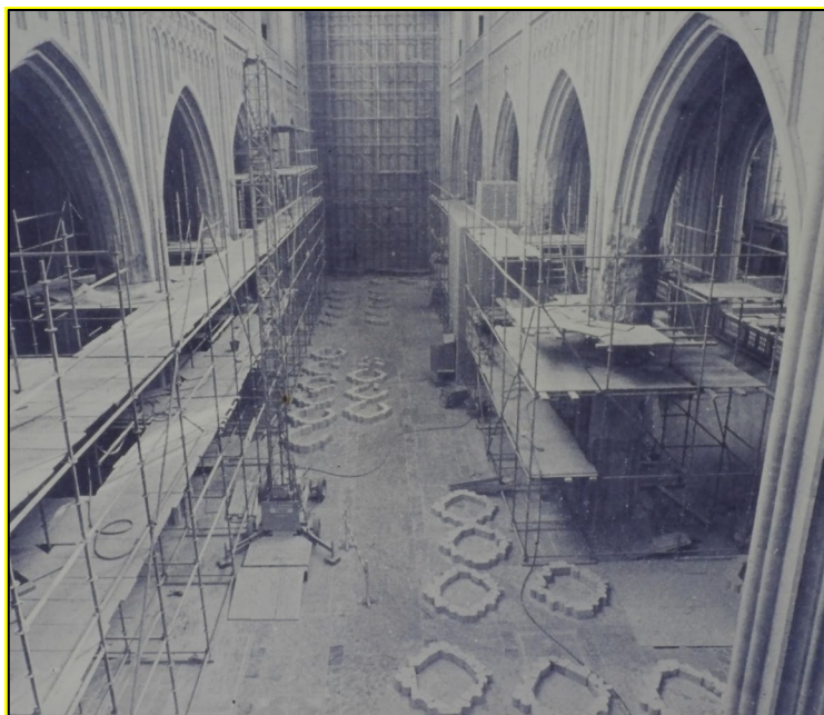
Figure 3. Interior of the Cathedral of Antwerp during the restoration of the pillars. The replacement stones are ready to be put back in place after the brick masonry core of the pillars have been injected with epoxy resin to provide it with sufficient carrying capacity to carry the load of the structure on each pillar. (Kinsbergen e.a., 1983, p. 31).
