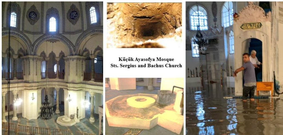
Figure 14. Küçük Ayasofya Mosque after a heavy rain
