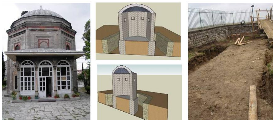
Figure 10. Retaining wall of the tomb at Yavuz Selim Mosque
