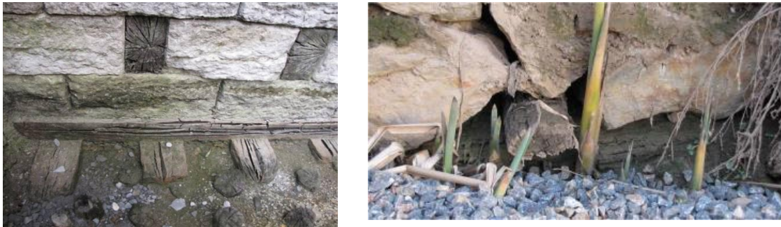
Figure 6. Wooden grillage of a Üsküdar and Sirkeci Byzantine chapels in Istanbul
