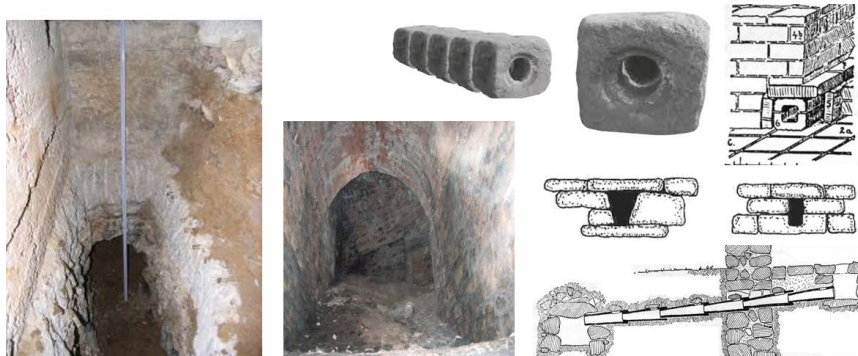
Figure 12. Discharge of underground water
