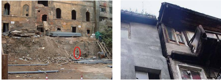
Figure 13. New construction beside a masonry building
