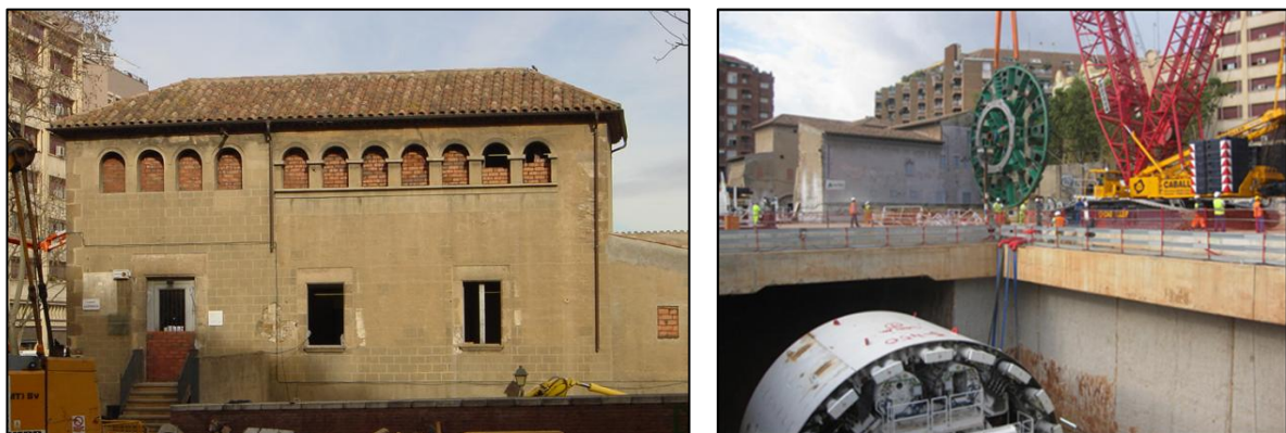
Figure 1. Left: Front view of the “Torre del Fang” building. Right: Rear view of the building with the tunnel and the assembling of the TBM.
