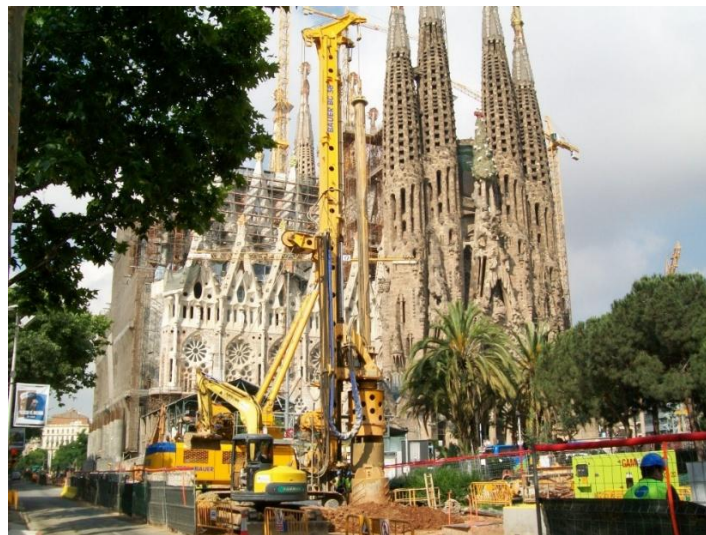
Figure 9. Construction of the pile wall along Mallorca street, close to the Sagrada Familia basilica.
