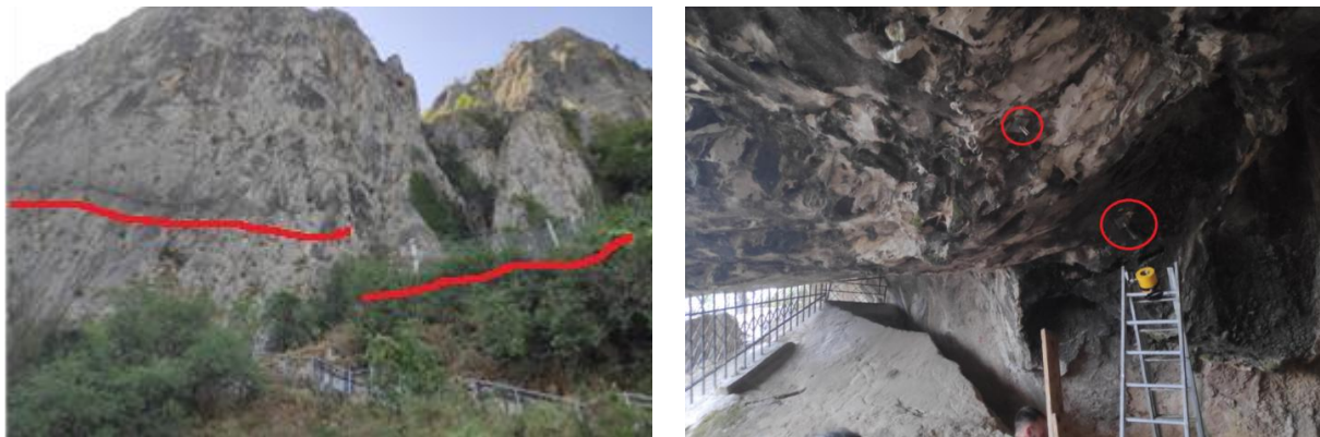
Figure 8. Left: The protective barrier above the entrance and the visitor walkway on the near-vertical slope. The protective barrier (6m; 5000kJ) above the ticket office and the visitor walkway is nearly hidden by the tree-line. Right: Anchors (AISI316; Ø27~28) on the wedge above the cave entrance (inside), right before non-destructive tests.
