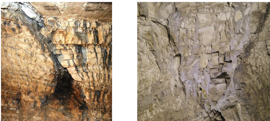
Figure 9. Pre-intervention view (left), and Post-intervention view during the 2026 inspection of the fault zone at Ch. 626 stabilized by pressure grouting (right).
