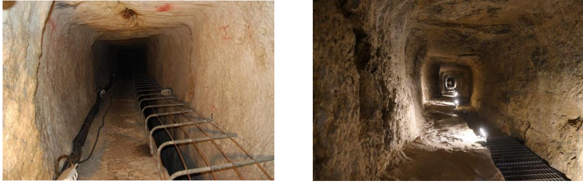
Figure 13. The pre-existing steel grill prior to the intervention at Ch. 568 (left). Installed structural grates during the 2026 inspection at Ch. 960 (right).
