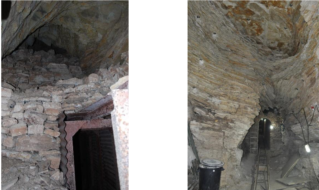
Figure 3. Pre-intervention sheltered walkway constructed by the DAI (left); the same location during installation of rock support measures after clearing (right).
