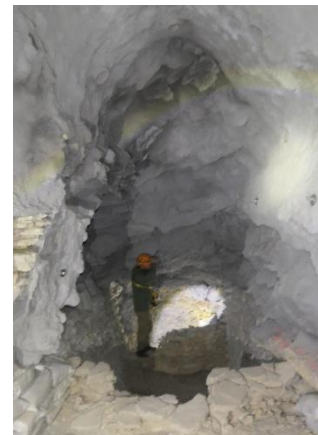
Figure 2. Cross section with the implemented support measures within the cavern above Roman lining (left). Pre-intervention rockmass condition in the cavern (middle). Post-intervention state during the 2016 inspection, displaying shotcrete, rock anchors, and dry concrete bags (right).
