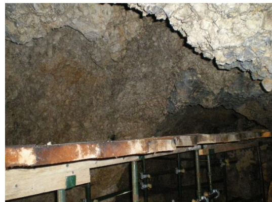
Figure 10. Design cross-section detailing the anchored stainless steel netting system between Ch. 999 and Ch. 1007. Pre-intervention view of the cataclastic rock mass of the section structure showing the temporary protection measures (right).
