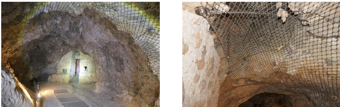
Figure 11. View of the installation of the support system during the 2026 inspection (left). Close-up detail illustrating the wire netting retaining detached rock fragments (right).
