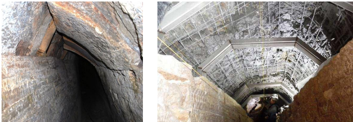
Figure 5. Distorted section between Ch. 130 and Ch. 136 prior to reconstruction (left). Representative view of the restoration process following the removal of the tholites (right).
