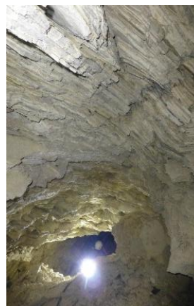
Figure 2. Cross section with the implemented support measures within the cavern above Roman lining (left). Pre-intervention rockmass condition in the cavern (middle). Post-intervention state during the 2016 inspection, displaying shotcrete, rock anchors, and dry concrete bags (right).
