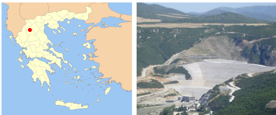
Figure 5. Location and downstream view of the Ilarionas Dam (REC Productions (kozan.gr))
