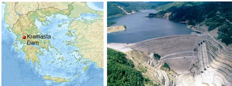
Figure 12. Location and view of the Kremasta Dam and reservoir (GCOLD)
