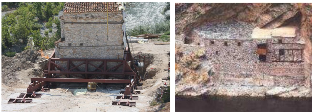
Figure 7. a. Moving the Katholikon on steel rails and b. The Skete of the Monastery of Osios Nikanor
