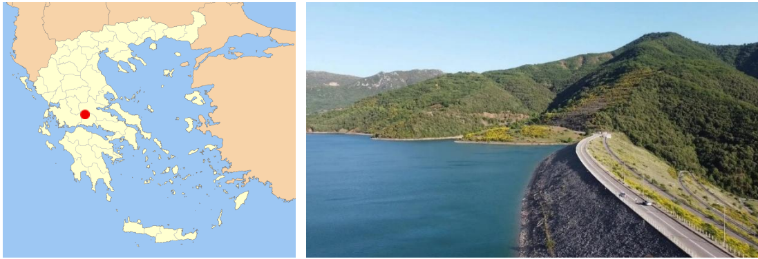
Figure 10. Location and view of the crest of Mornos Dam (Michanikos, 2023)
