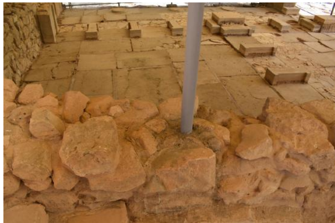
Figure 5. Steel column founded directly on an ancient wall of the Royal Chambers via surface contact.
