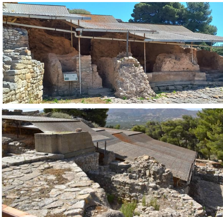
Figure 3. Steel frame canopies with corrugated asbestos-cement sheet coverings over the Old Palace complex: view from west towards east (top) and from north to south (bottom).
