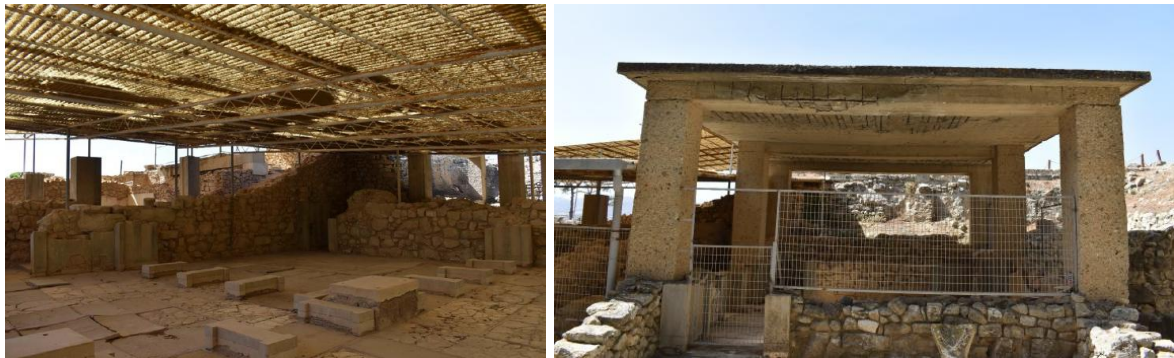
Figure 2. Shelter canopies covering the Royal Apartments: partially a steel frame canopy with corrugated plastic sheet coverings (left) and reinforced concrete canopy of smaller dimensions (right).
