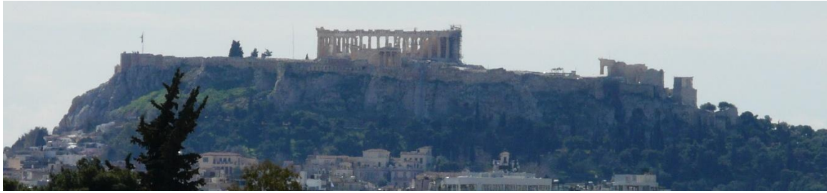
Figure 1. Typical view of the north side of Acropolis as viewed by millions of Athenians and visitors of Athens. Erechtheion in the foreground, Parthenon behind it and Propylae on the right attract most of the interest, but it is the circuit walls (even from the north side as in the photograph -shorter than those on the south or western side) that frame the citadel and form the Athens skyline.
