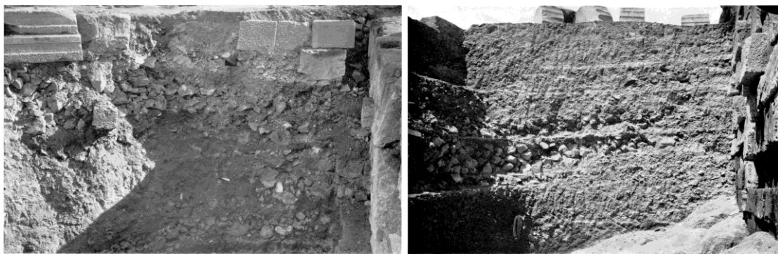
Figure 3. Views from the 19th century great excavation demonstrating the macroscopic nature of the earthfill (left) and the big height of the free standing vertical faces of the excavated earthfill (right).
