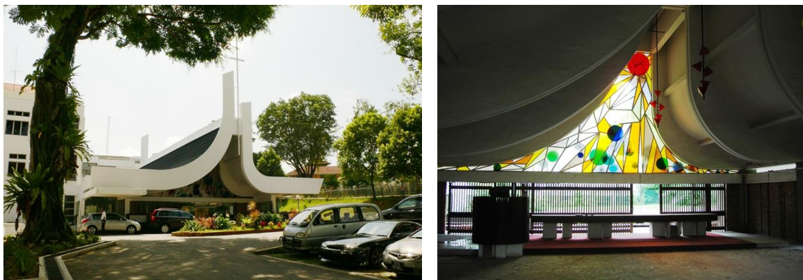
Figure 4. Former Trinity Theological College Chapel (Urban Redevelopment Authority, n.d.-b)
