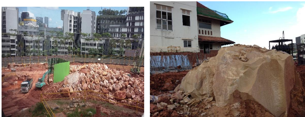
Figure 6. Sandstone boulders of various sizes exposed during excavation
