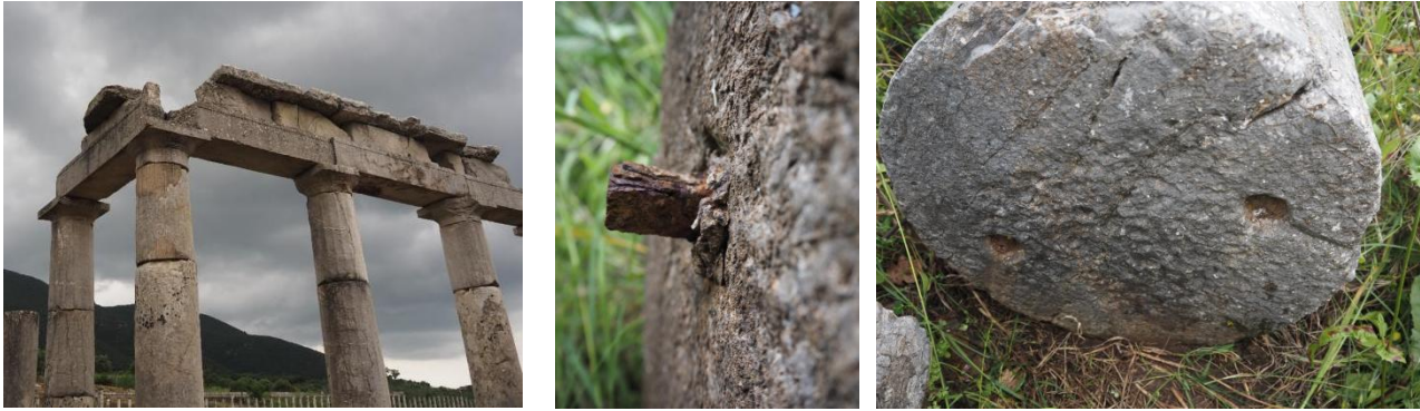
Figure 5. The Gymnasium, in the archeological site of Ancient Messene: The construction of the corner and the form of the epistyles (left); Drum, the iron connector can be seen (middle); Drum with grooves and channel for the lead pouring (right).
