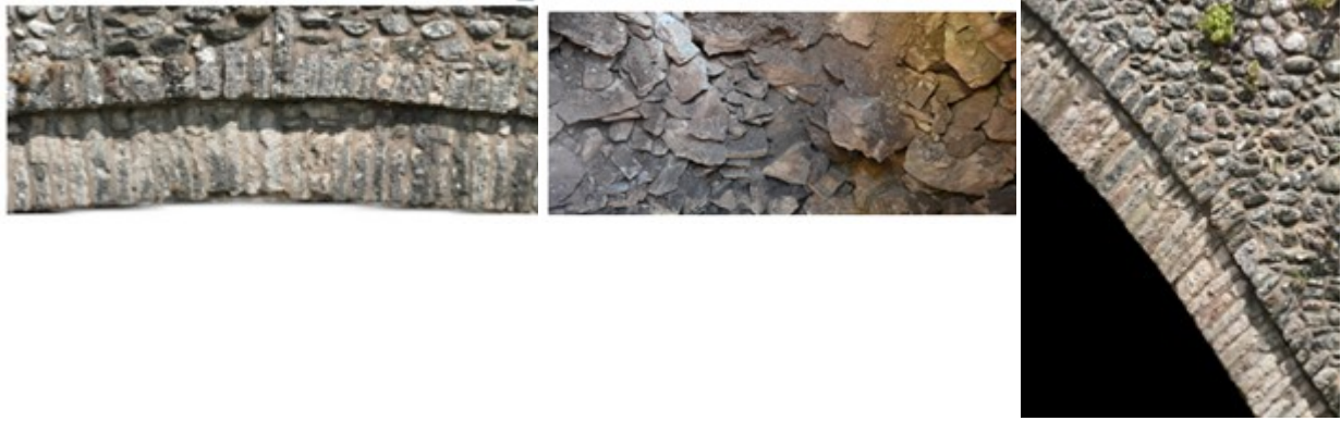
Figure 5. Characteristic segments of the Pyli Bridge: arch, fill, and spandrel drum.
