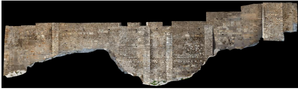
Figure 3. Later stonework with mortar (reconstruction) of the eastern section of the Circuit Wall of the Acropolis (YSMA, 2020).
