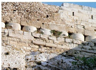
Figure 1. Characteristic area of the north side of the Circuit Wall, where the ancient wall and later phases intertwine
