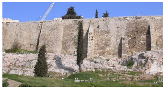
Figure 2. Characteristic area of the south side of the Circuit Wall, where only later phases are visible
