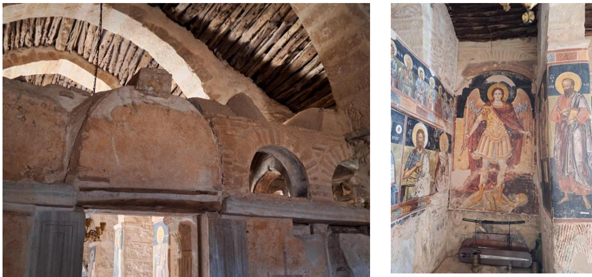
Figure 4. Interior of the monument with visible timber roof (left) and painted decoration with frescoes of the 18th century, from the school of Georgios Markos (right).
