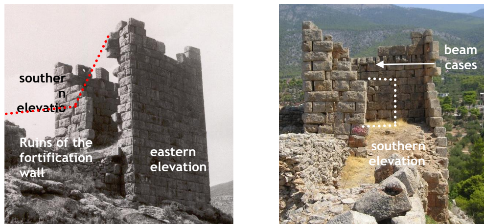
Figure 1. The southern & eastern elevations of the tower in 1933 (courtesy of the German Archaeol. Inst., Athens). In dotted line: the missing fortification wall (left). The tower after collapse of the S.E. corner and eastern elevation (1981)-in white dotted line the entrance to the first level is shown (right)
