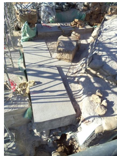
Figure 11. The deep foundation under construction (view from the east) (left). The pile cap of the eastern elevation before the anastylosis and, in the background the western one (right).
