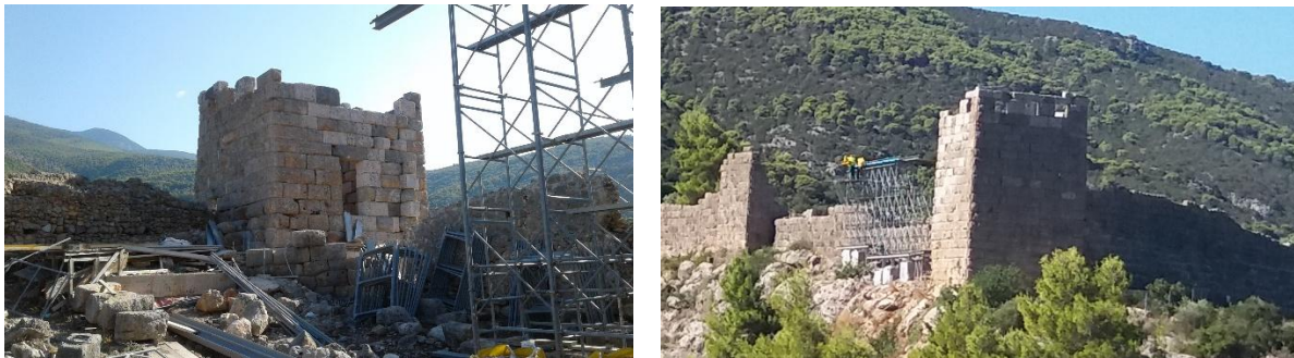
Figure 12. The restored south and western elevations from the interior of the acropolis (left). The restored eastern and northern elevations (right)
