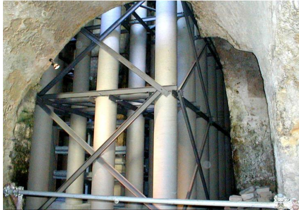
Figure 5. Emergency reinforcement by concrete pillars (1991 – Pierre Regaldo Saint-Blancard)
