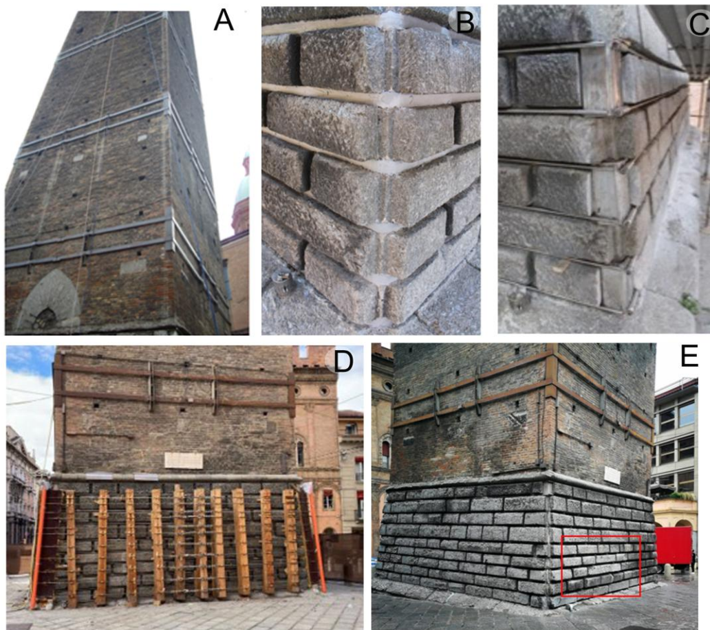
Figure 3: A) Perimeter belts confining the masonry wall; B) Passive confinement of the tower basement obtained through FRCM belting along horizontal joints of the selenite cladding, C) Active confinement of the tower corners by insertion of post tensioned stainless steel bars and corner stainless steel plates; D) Active confinement of the cladding through a funicular belting of the tower base. E) Bowing of the east side of the selenite cladding. Photos from A to D modified from de Miranda et al. (2025), photo E from Dallavalle et al. (2022).
