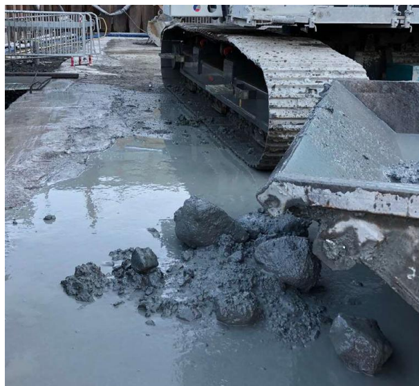
Figure 4. Example of large boulders extracted from the moraine layer during diaphragm wall excavation.
