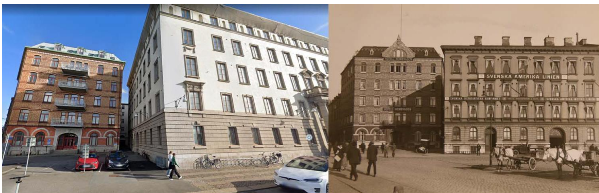
Figure 7. Building 13.12: comparison between recent status (left) and historical status at 1920 (right).
