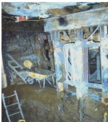
Figure 2B. Picture of the underpinning corridor at Helen Street. All the concrete piers were jacked.
