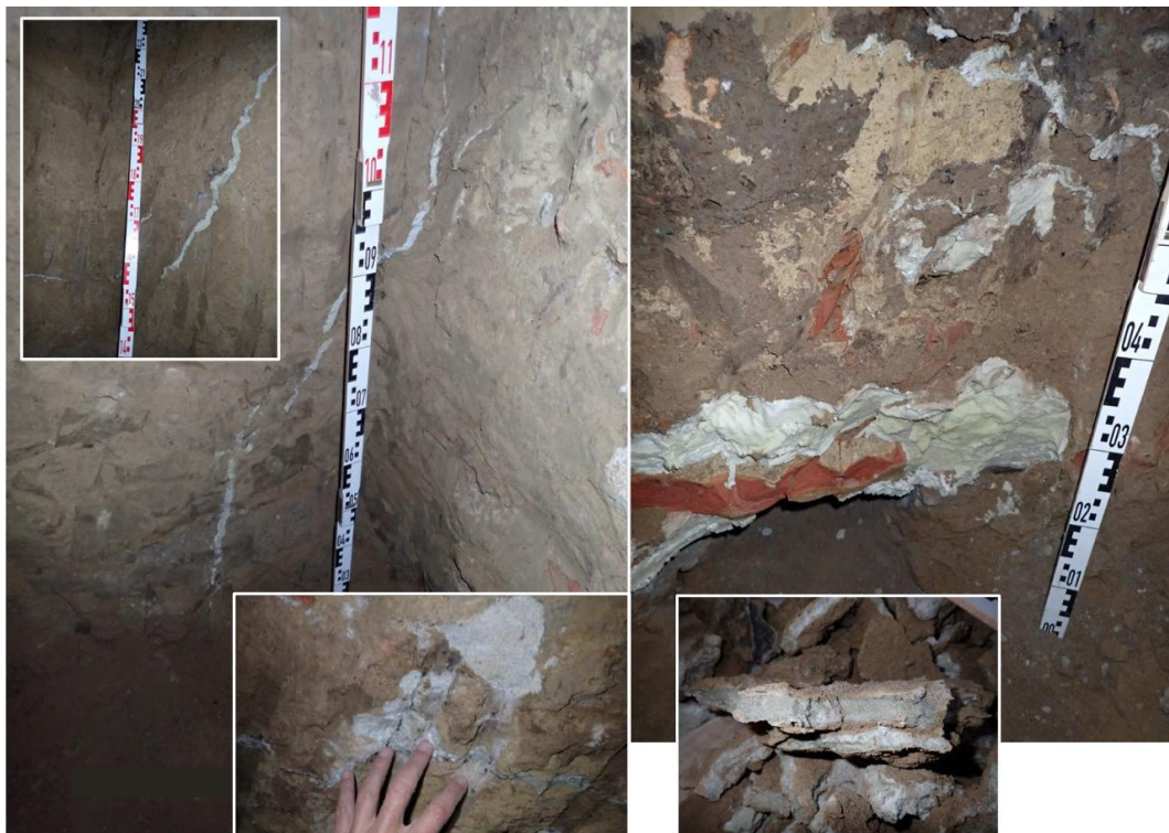
Figure 5. Images of the soil beneath the building foundation after the injection of expanding polyurethane resin
