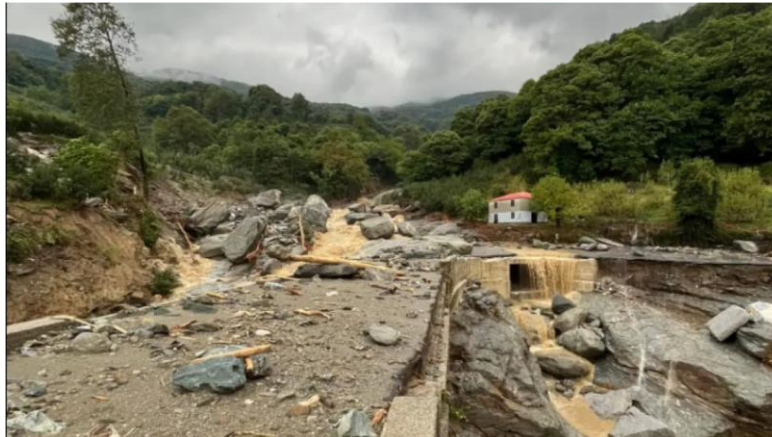
Figure 1: Damage caused in Zagora by landslides due to heavy rainfall
