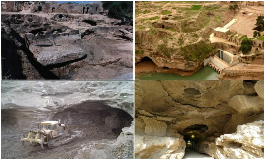
Figure 4. Front view of Daryun canal before (left) and after (right) rehabilitation works (below).
