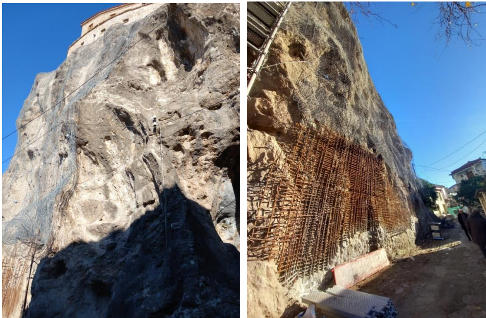
Figure 8. (a) Installation of anchored wire mesh, (b) filling of voids with cement at the base of slope in overhanging areas.
