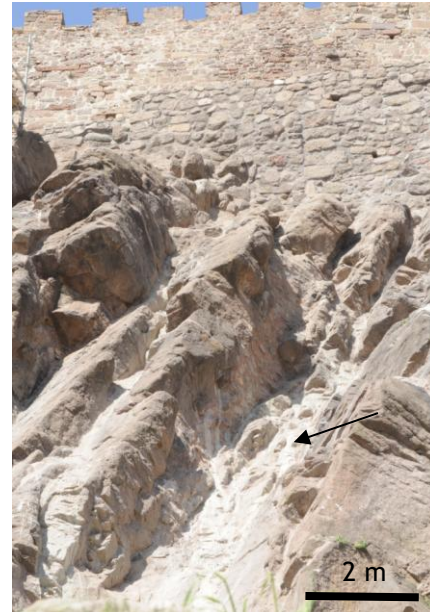
Figure 4. (a) Drawing detail of void filling with concrete and stone wall facing to support overhanging blocks. (b) constructed filling shown with arrow, example from Mythemna Castle.
