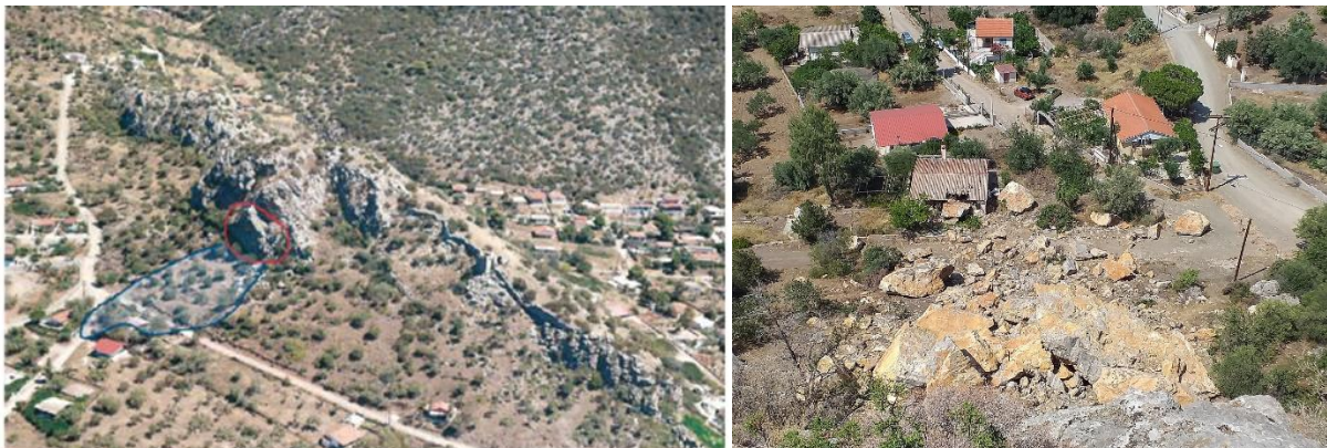
Figure 12. (a) Aerial photograph showing the location of the 2019 rockfall detachment and the area of rock blocks deposition b) Rockfall event impacting houses.
