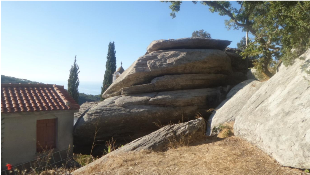
Figure 9. Gneiss rock mass sliding on foliation plane and impacting a historic church. The church is downslope behind the rock block.
