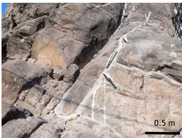
Figure 3. Sealing open joints in basaltic rock mass at Mythemna Castle, Lesvos Island.
