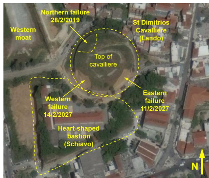
Figure 2. Close in on the area of the St Dimitrios Bastion indicated by the rectangle in the dashed yellow line in Fig. 1. The bastion itself, the cavaliere and the locations of the 2017 & 2019 failures are indicated.
