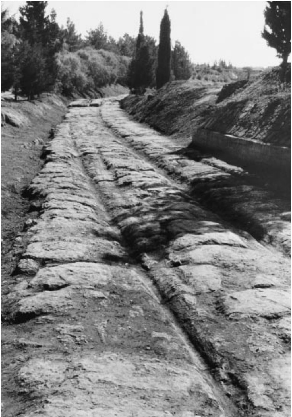
Figure 11. The Diolkos in September 1978. The tracks and side tracks are clearly visible. The stones to the right are part of a modern supporting wall. (Photo: Author)
