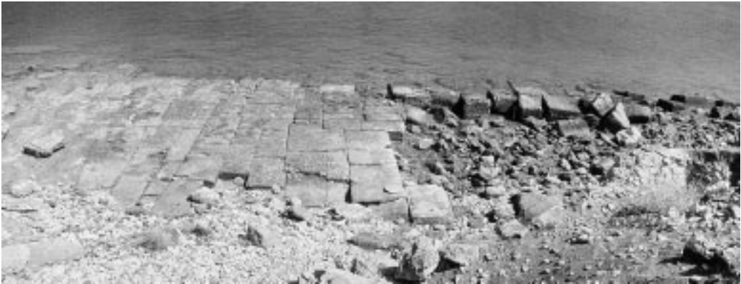
Figure 1. The western termination of the Diolkos next to the Corinth canal in September 1981 (sector A). This so-called mooring place has suffered from the wash of passing vessels. Since the photograph was taken, some of the carved stones have slipped into the canal. There are fewer stones in the group on the right. (Photo: Author)
