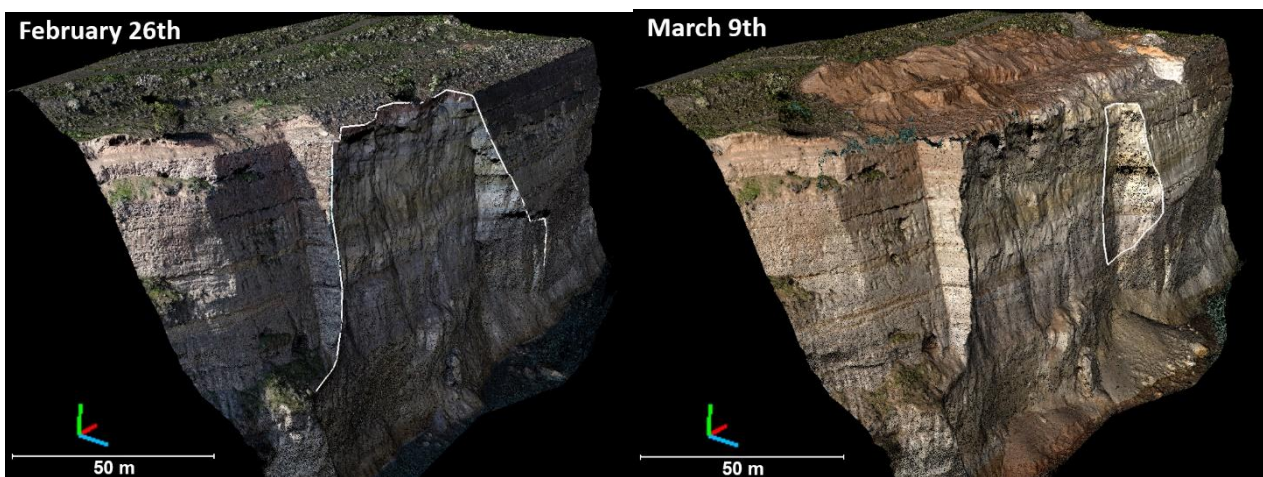
Figure 3. Point cloud of slope failure of Corinth Canal on February 26 th and March 9 th from Pix4D.
